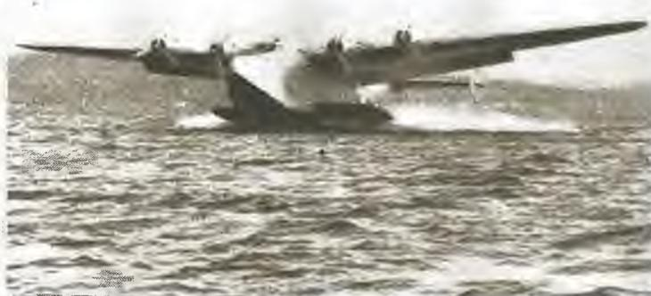
The 41 1/2-ton Boeing Clipper lands on Lake Washington, Seattle, after a test flight. Note the large wing flaps, lowered to decrease landing speed.
