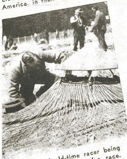
Safety valve of old-time racer being inspected before inflation for race.
